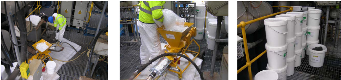
Pictures showing pumpable mastic in 20kg shipping containers and pump working space
