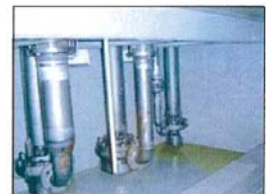
ISOPur BCA Treated Gas Turbine
