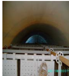
Inside a stack before
